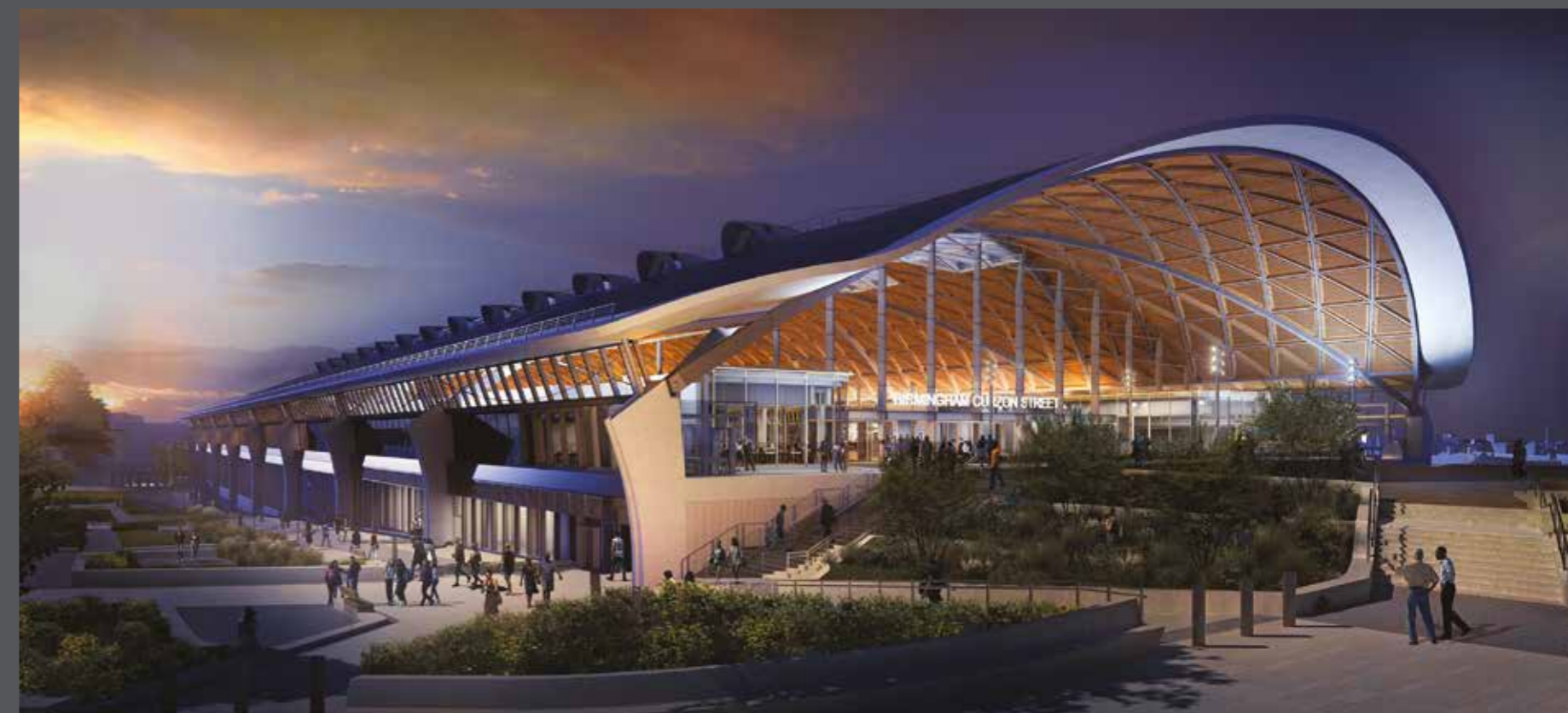
HS2 - BIRMINGHAM CURZON STREET STATION (BIRMINGHAM)
